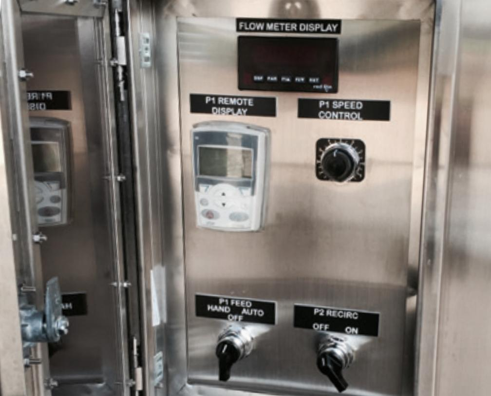
The manual electrical control panel is easy to use and NEMA 4-certified.
